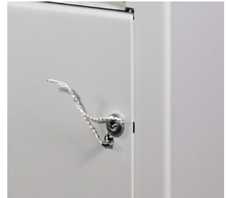
Ready for sealing.
