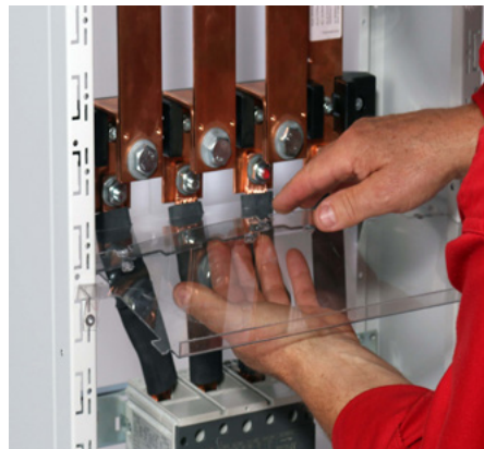
Put together the chips of the 2 plates and fasten the covering to the platform.
