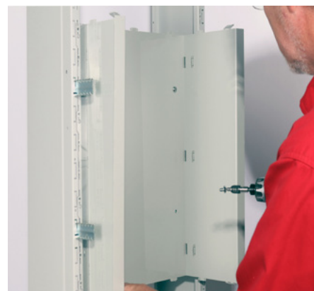
Then fasten to the platform in the 2 coverings.
