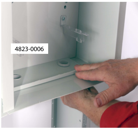
Mount the support plate - remember that the membrane should go through both plastic layers.
