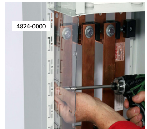
Side coverings are mounted in both sides.
