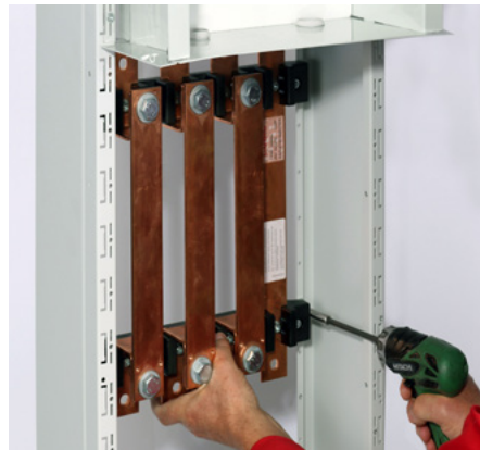
Transformerfelt skrues fast.
