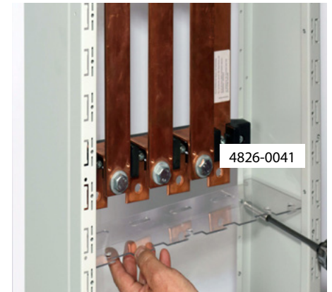
Vandret afdækning monteres under transformerfelt.
