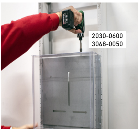
The covering is screwed together with washers and screws.
