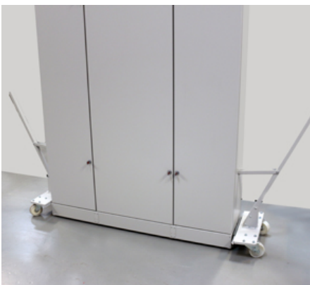
The panel can now be moved in to place
