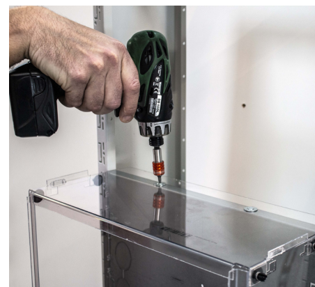
Holes must be drilled in the metal plate for mounting of screws for fastening of top and bottom.
