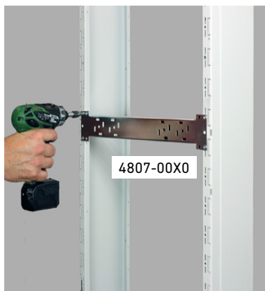
Busbar carrier to be screwed on the platform.
