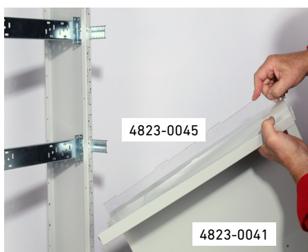
Coverings are clipped on the house.
