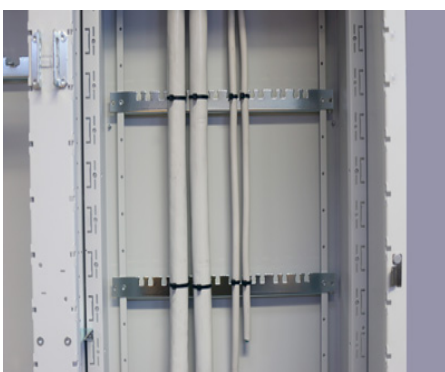
Wires fixed with cable tie.
