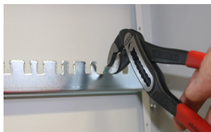
For easier mounting of cable tray, bend a pin out in both sides of the cable support.
