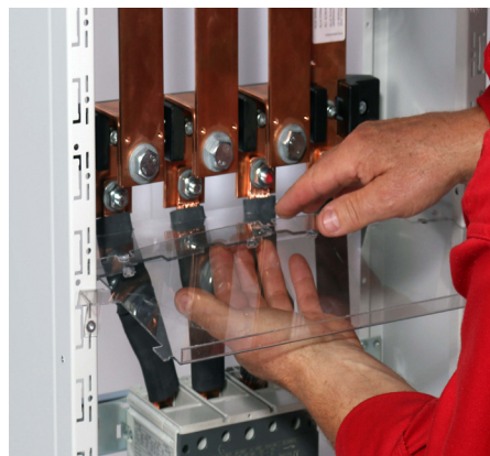
Put together the chips of the 2 plates and fasten the covering to the platform.
