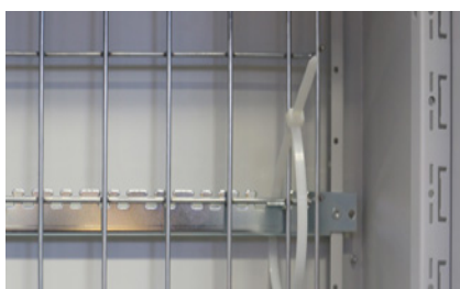
Cable tray is then mounted with cable ties. Use 2 cable ties \geq 535Nm per. cable support.
