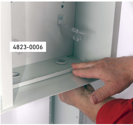
4823-0006 Mount the support plate - remember that the membrane should go through both plastic layers.
