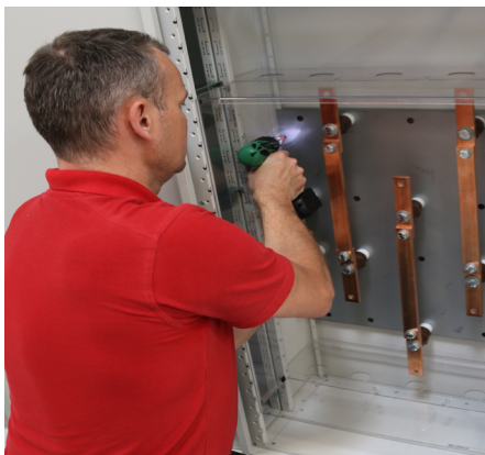
Mounting plate is mounted.
