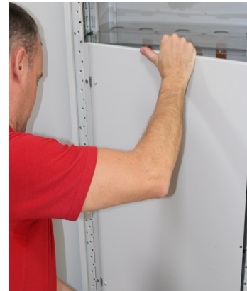
Front with swing frame is mounted.
