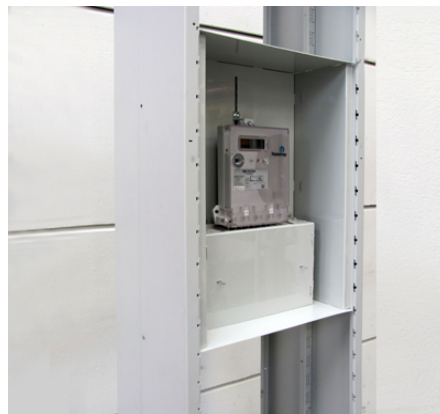
It is covered, and is now ready for meter and seal.
