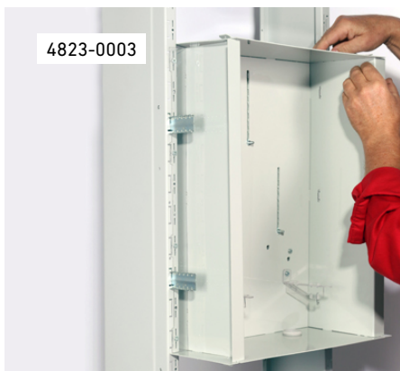
Top and bottom are clipped into place.
