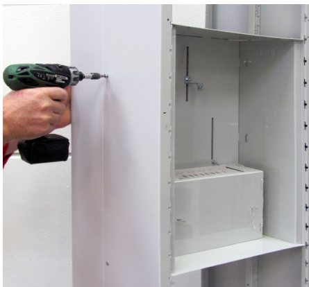
Sides for the platform are mounted with screws.
