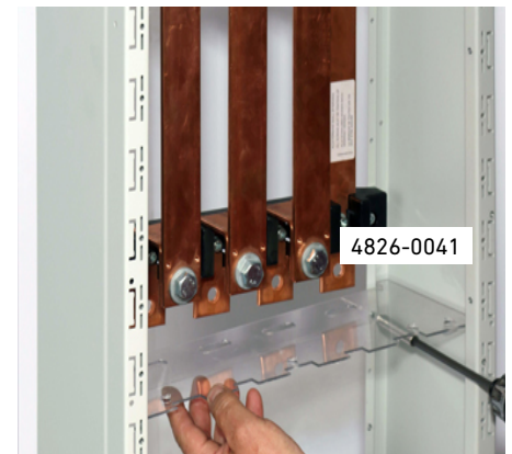
Vandret afdækning monteres under transformerfelt.
