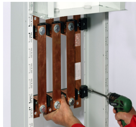
Transformerfelt skrues fast.
